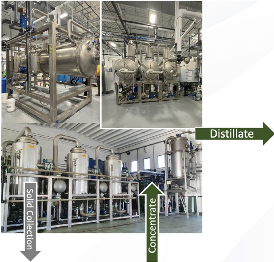
Figure 2: An overview of the major components that define a ZLD, closed-loop, water recycling system in a fab.
