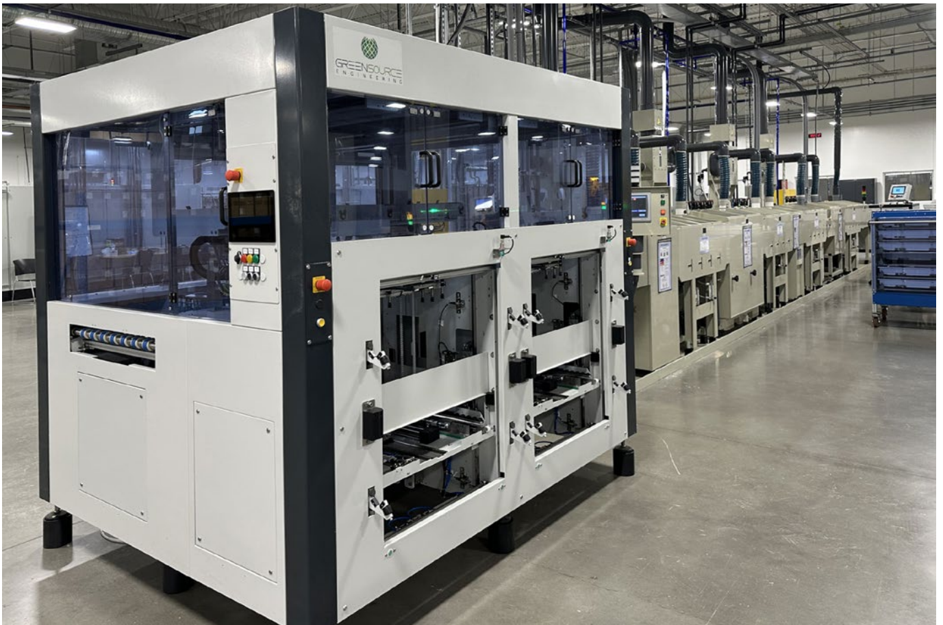
From left: GreenSource Engineering (GSE) double loader, photoresist strip line, GSE unloader.
