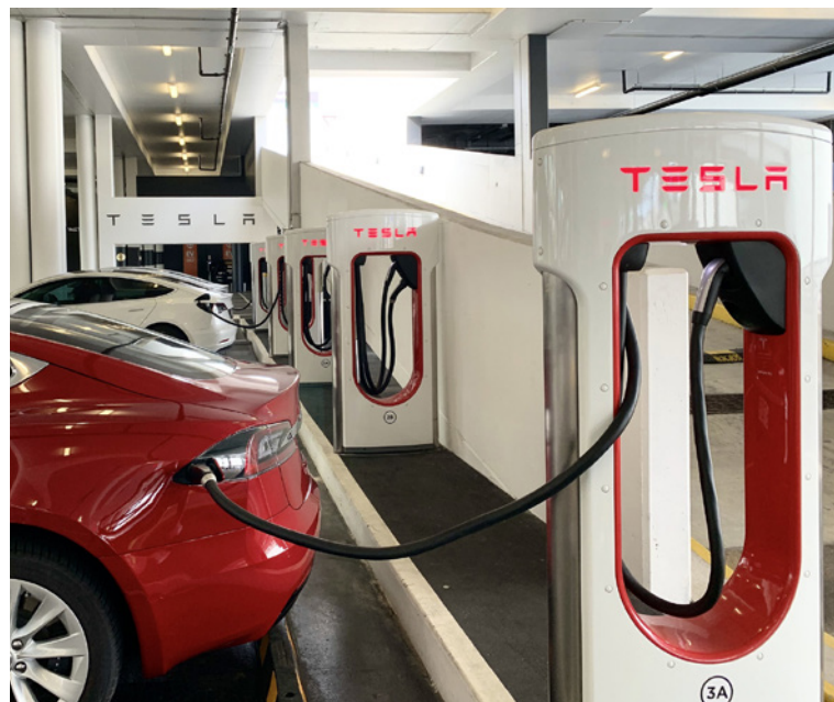
Figure 2: Level 3 DC fast charger. (Source: Creative Commons, Kgbo, 2020)
